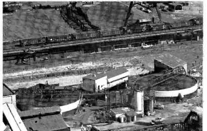
As part of Republic's water quality control program, additional facilities are being constructed at #5 and #6 blast furnaces to permit reuse of treated water.
