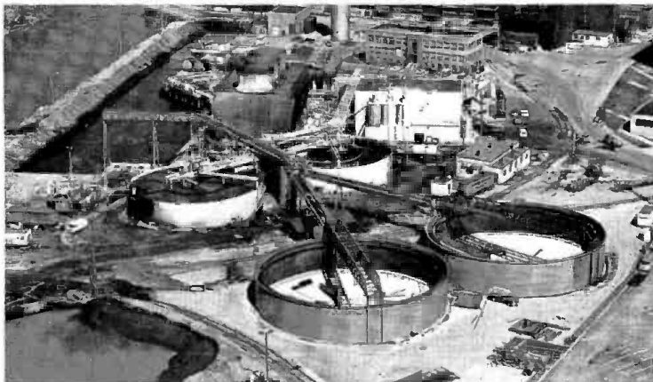
Water Treatment Plant at Republic's hot and cold strip mill complex recycles more than 100 million gallons of water daily. Original cost: $18 million Additional water clarifiers: $6 million
